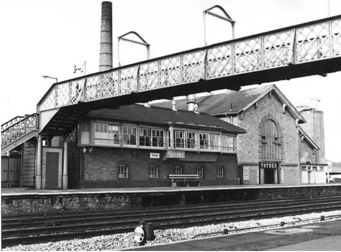
Totnes Signal Box and the original Victorian wrought iron footbridge (before it was replaced after being hit by a crane engaged in track renewals in 1987)
