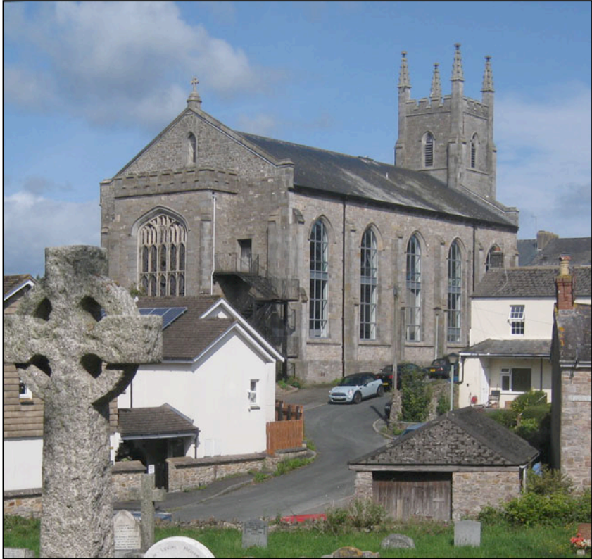
St John's seen from the burial ground across Weston Road
