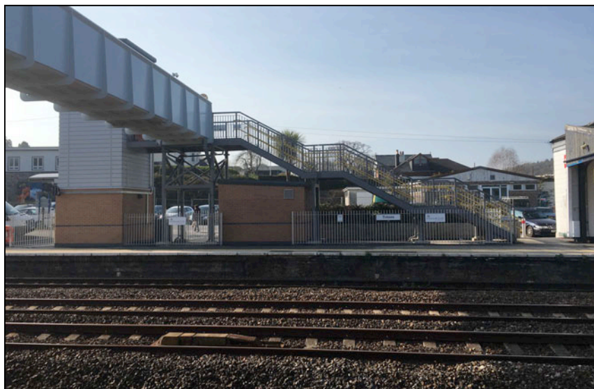
New footbridge and lift on platform 1
