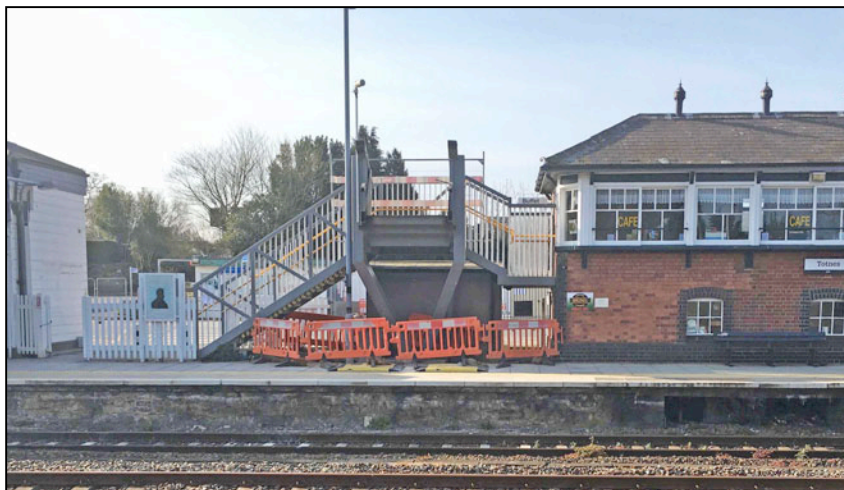
Remains of the old footbridge on platform 1
