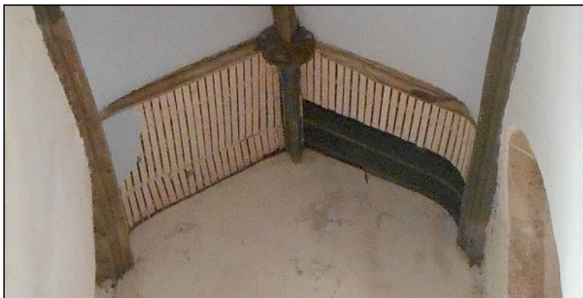
The south aisle and below detail of the fallen plaster
