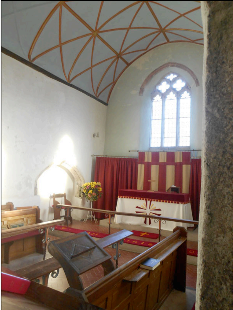
The nave and altar showing the moulded plaster wagon roof
