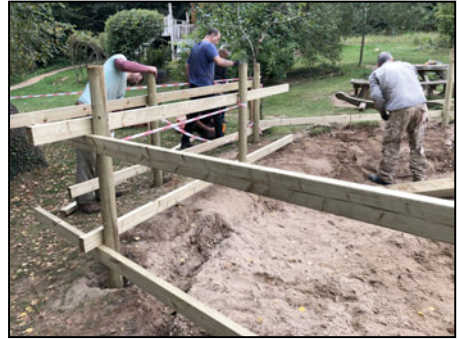
setting the posts and fixing the rails
