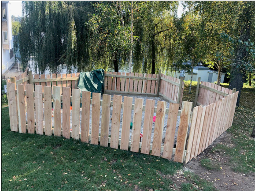
Almost complete – tops of cladding still to be shaped
